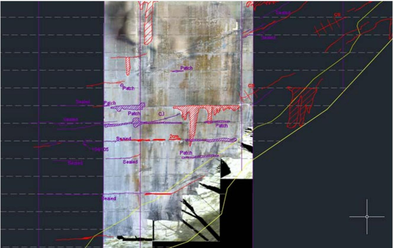
A section of the defect report, overlaid on one of the project's high-resolution orthoplanes.
