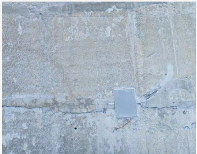
One of the albris's individual images, featuring the metal plate of a crack gauge (measuring 46 x 34 cm / 18 x 13.4 in). Each photo was captured 3.7 metres away from the face and covers a surface region of 4.6 x 3.5 m (15 x 11.5 ft).
