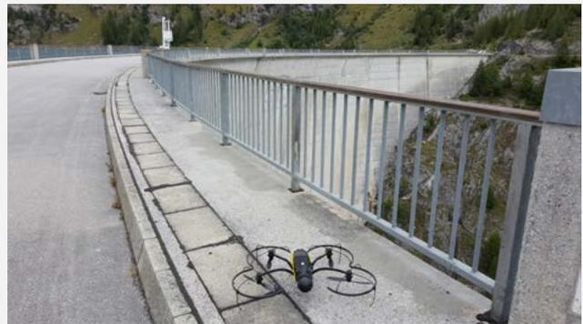
*The senseFly albris on the road atop of the dam's downstream face, ready to go to work.*
