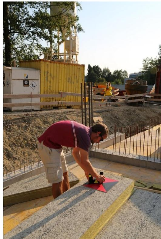
Figure 3 – A small reflective target was used to measure the ten marker locations with the total station.
